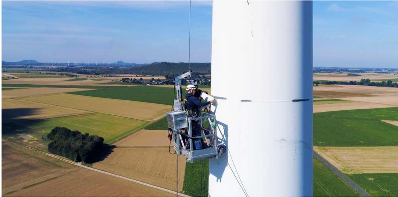
currently being used in a pilot project on a North Sea transformer platform. It is a high-performance film called RENOLIT CP Advanced that fundamentally changes the fight against corrosion. The innovation lies in its ingenious structure: a high adhesive layer thickness ensures reliable adhesion, even on rough, uneven surfaces. After cleaning and removing corrosion, the film can be applied directly – without primer, as this is already integrated, as is the anti-corrosion effect.
