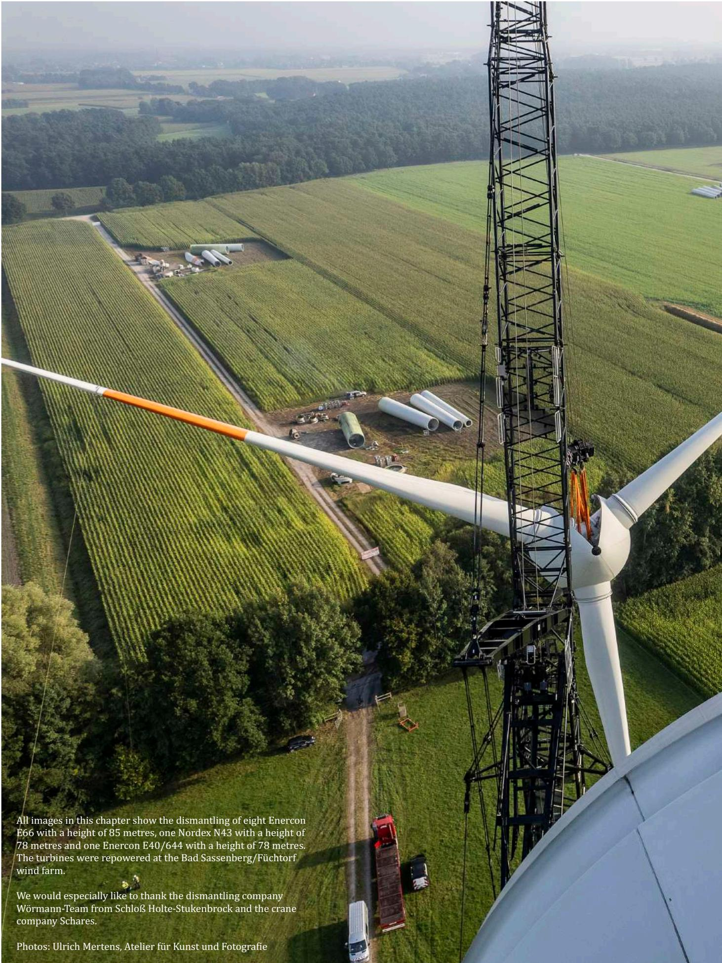
All images in this chapter show the dismantling of eight Enercon E66 with a height of 85 metres, one Nordex N43 with a height of 78 metres and one Enercon E40/644 with a height of 78 metres. The turbines were repowered at the Bad Sassenberg/Füchtorf wind farm.
